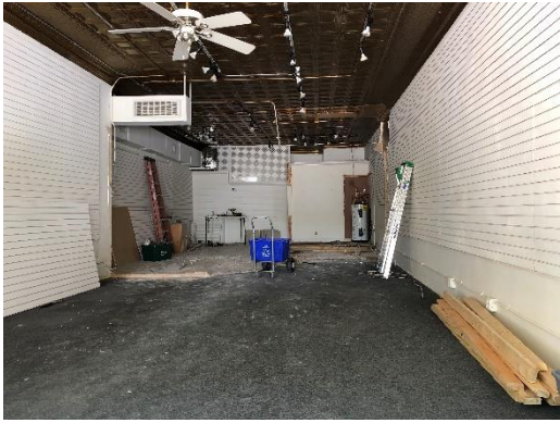
Figure 5 Walls Taken Down
