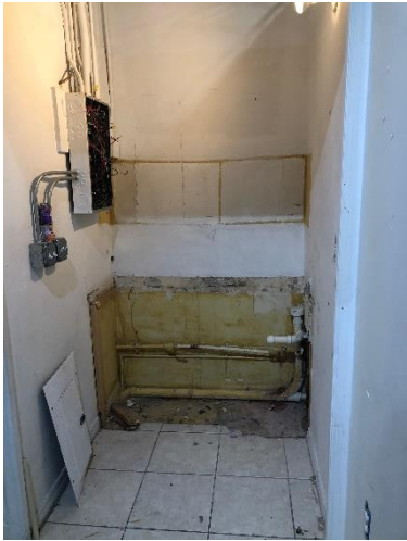
Figure 7 Kitchen Cabinets Had to Be Removed
