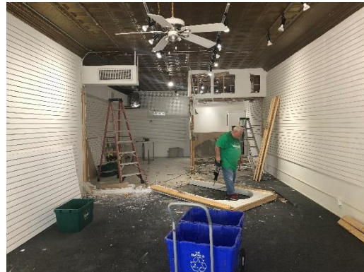
Figure 2 Interior Walls Removal
