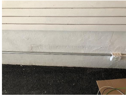
Figure 8 Conduit That Will be Removed
