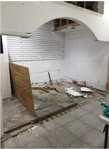
Figure 1 Alcove Floor Removal
