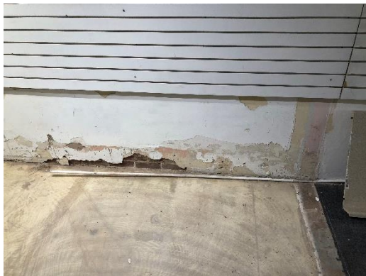
Figure 9 Condition of Walls That Will be Covered with Plywood
