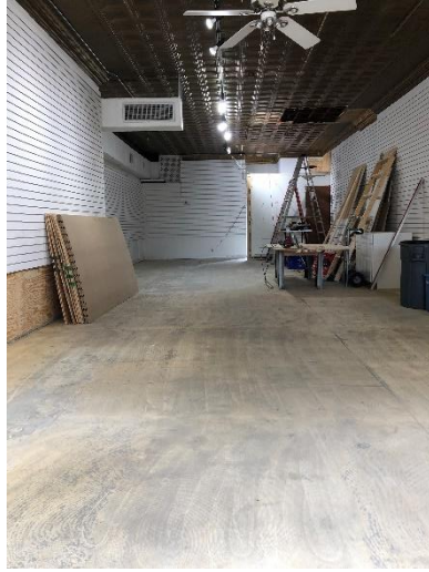
Figure 6 Old Flooring Removed
